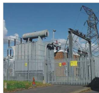
Engineering Procurement & Construction (EPC)
